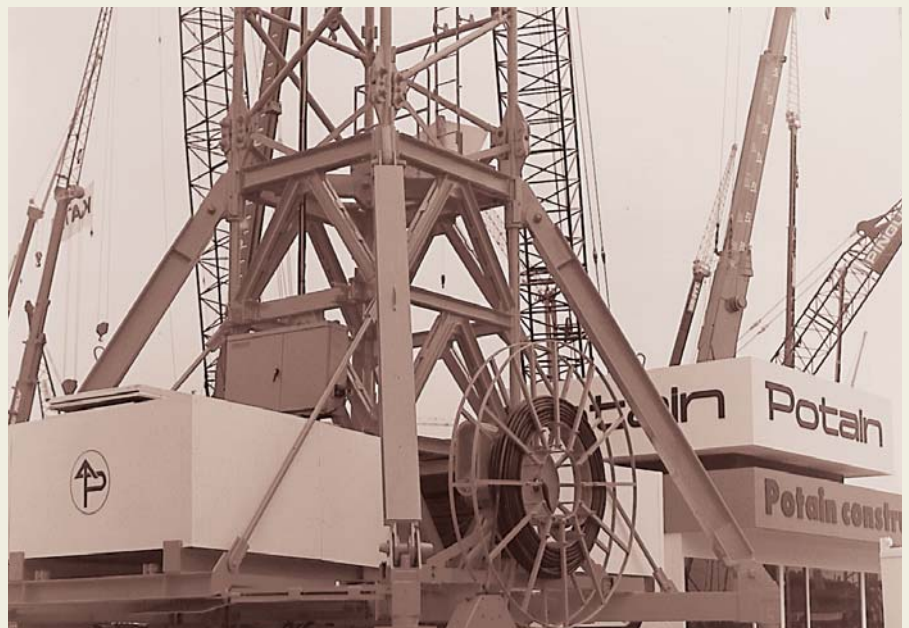
Potain tower crane - 1966.
