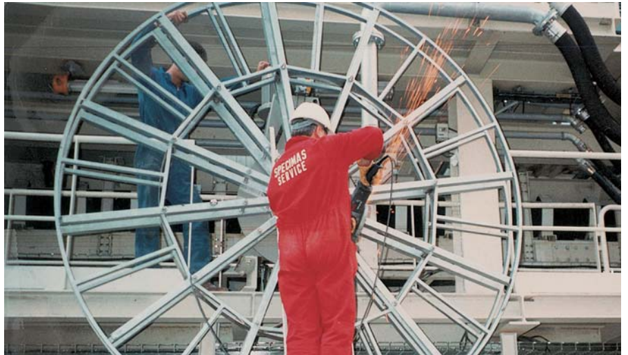
The commissioning of a giant hose reel for Madrid metropolitan tunnel drilling.
