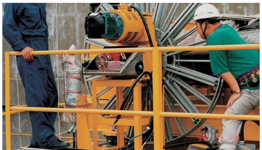
A cable reel being commissioned in Korea for a compost plant application.
